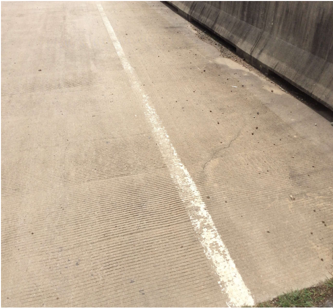
PHOTO 1 Description The driving surface of the deck has sealable cracks.
