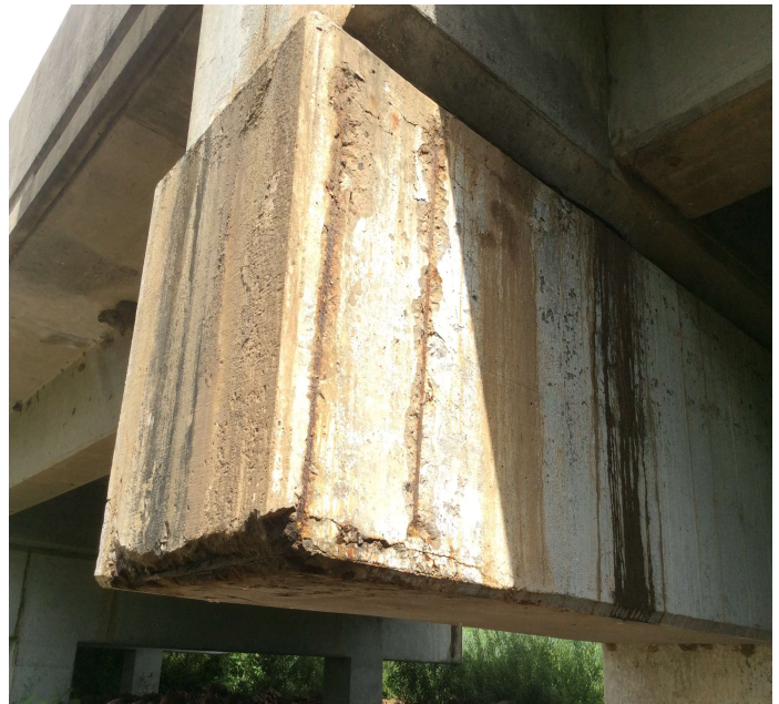
PHOTO 2 Description The Rt end of Bent 4 cap has shallow 24" long spalls with exposed reinforcing steel (stirrups). Exposed reinforcing steel has active corrosion with initial section loss at this inspection.
