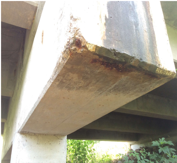
PHOTO 1 Description The Lt end of Bent 2 cap has delaminated areas with cracks and rust stains in the end of caps.
