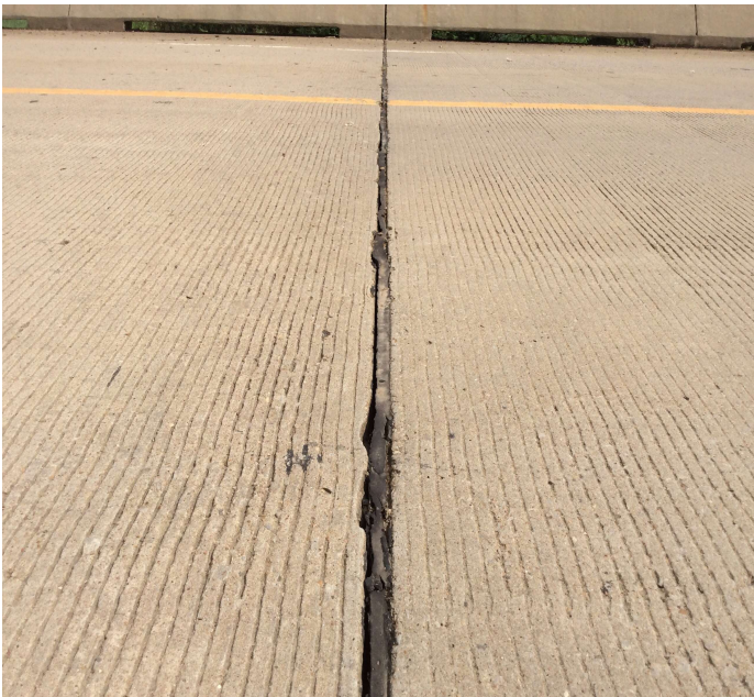
PHOTO 1 Description The compression deck joint seals are deteriorated and leak water on the substructure.
